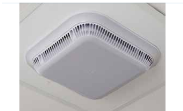
RAU5x (including external antenna) Mid-Mountable Installation | Figure 4
